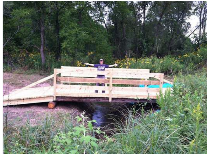
Amy Staffen on the new bridge at Kalscheur Savanna. Photo by Kristin Westad
