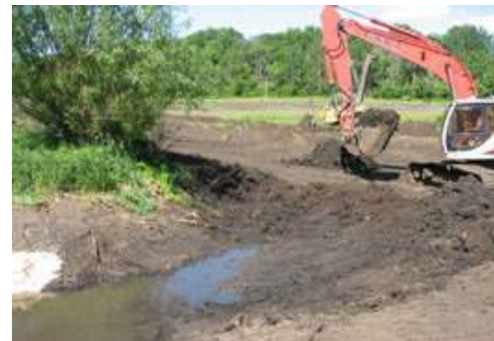
Removing post-settlement sediment from floodplain. Photo by Peter Ziegler
